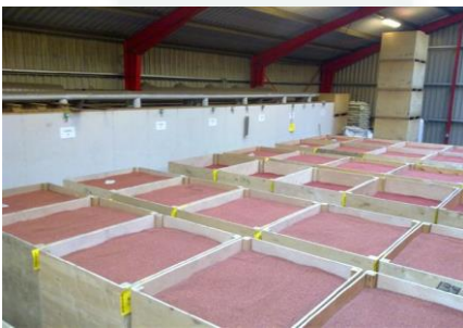
Existing installation for drying treated seed in boxes in 10 sections/lines.
