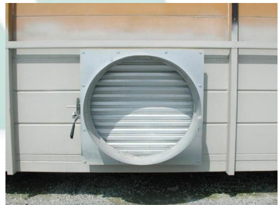
A modulated motor controlled valve would be installed in front of the air opening.
