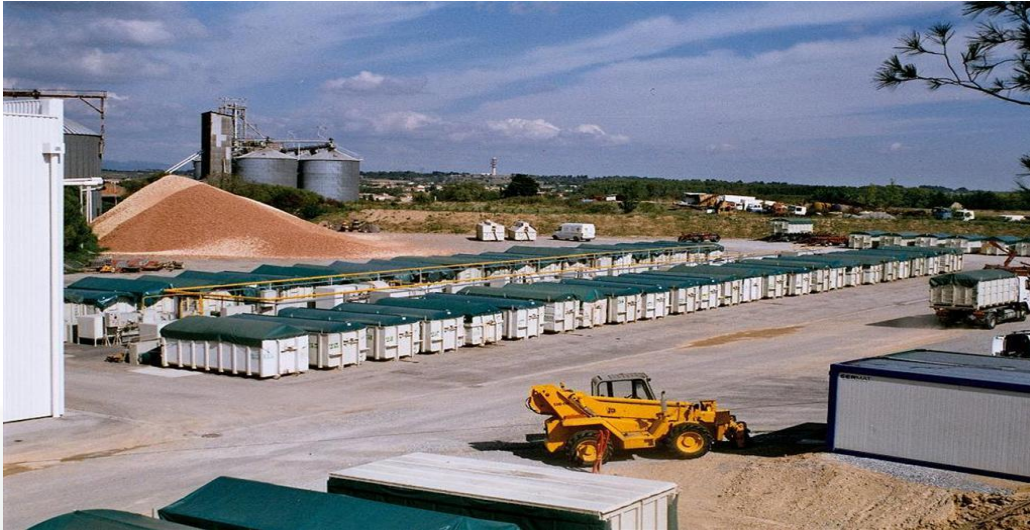
Overview of drying systems with containers
