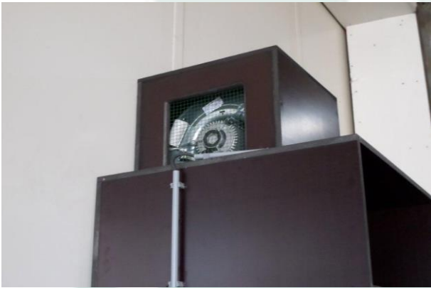
Centrifugal fan for extracting conditioned air to blow through the seed.
